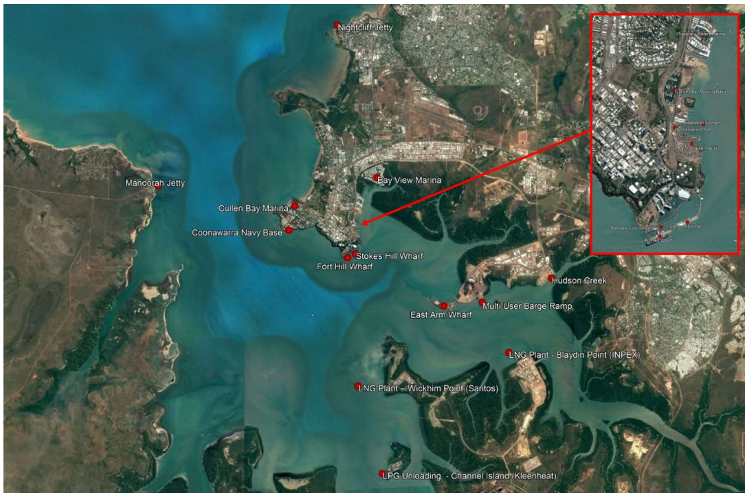
Figure 3.3 Port of Darwin Infrastructure
