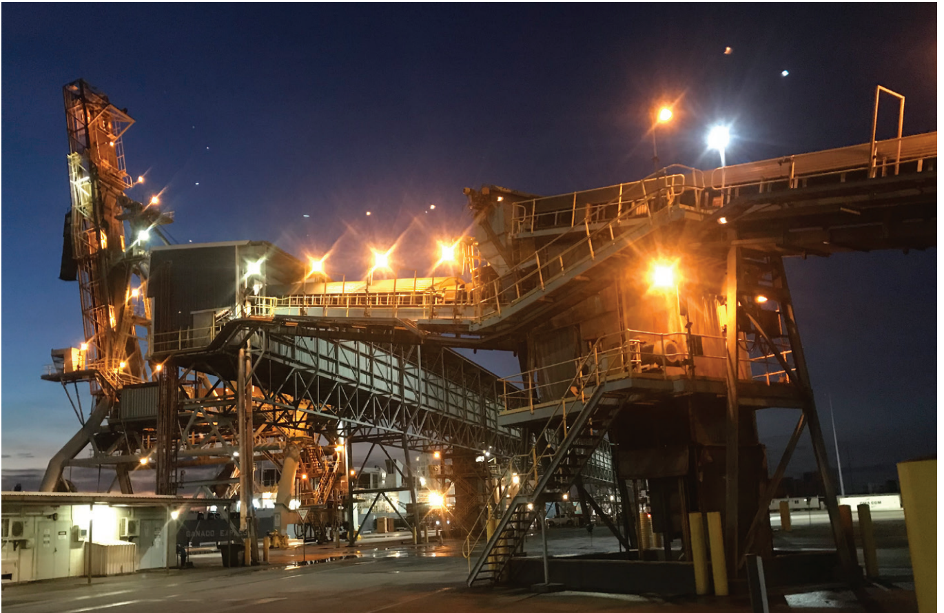
Bulk materials loader at East Arm Wharf
