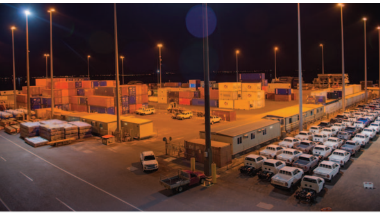
Darwin Port container storage yard
